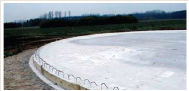
Reinforced cast in-situ concrete base
