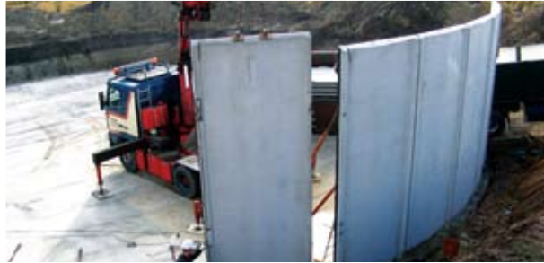
Fast track installation
